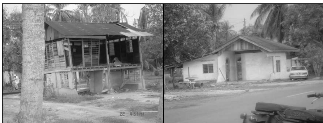
Figure 1.3: Houses in Kuala Muda, Kedah destroyed by the Andaman tsunami waves
