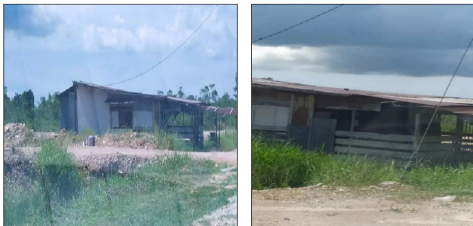
Figure 1.1 Temporary Housing Facilities in Jalan Kelupu, Bintangor, Sarawak
