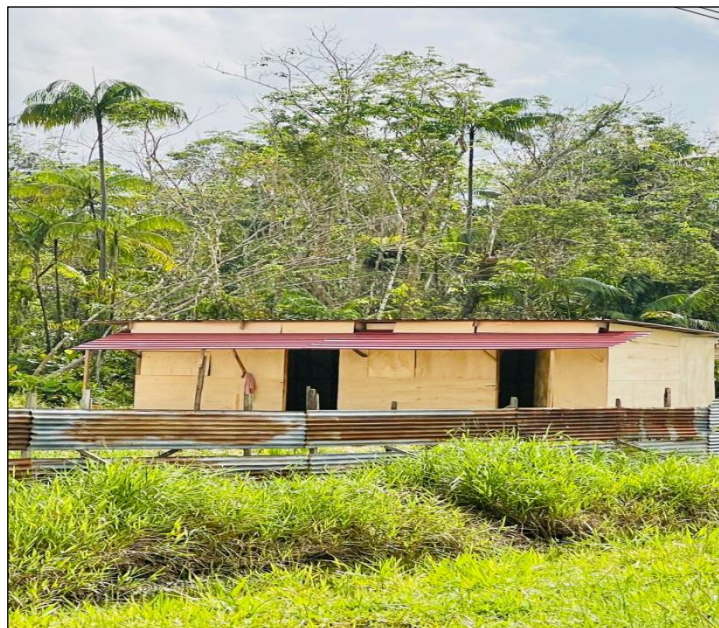
Figure 1.3 Temporary Housing Facilities in Sarikei, Sarawak
