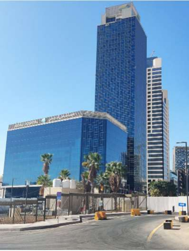
Figure 1.2 Larger glass sections Al-Abdali Hospital
