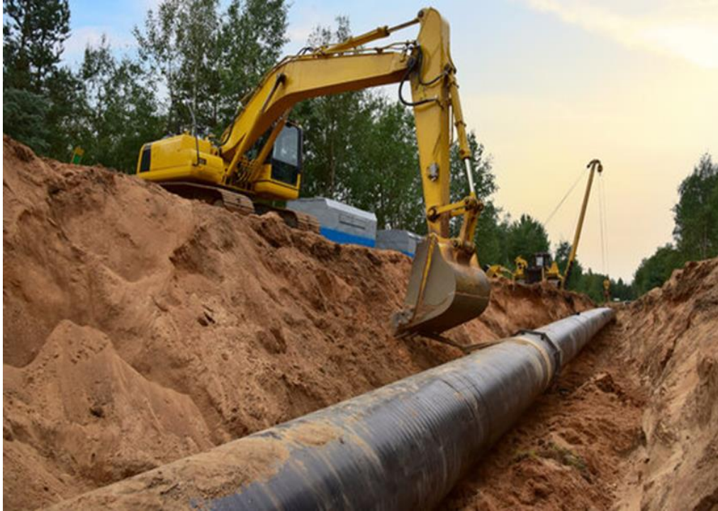
Figure 2 : Installing underground metal pipe
