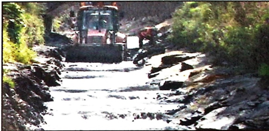
Figure 2.6: Canalization and related works (DID, 2010)
