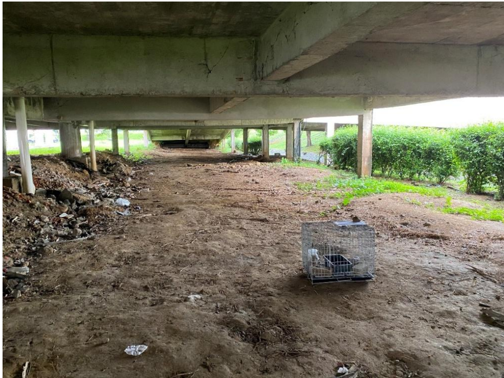
Figure 3.2 Control sample situated in the basement car parking area under the front entrance ramp of the PPSK building
