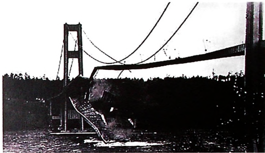
Figure 1.1: Failure of Tacoma bridge (Wikipedia, 2008)
