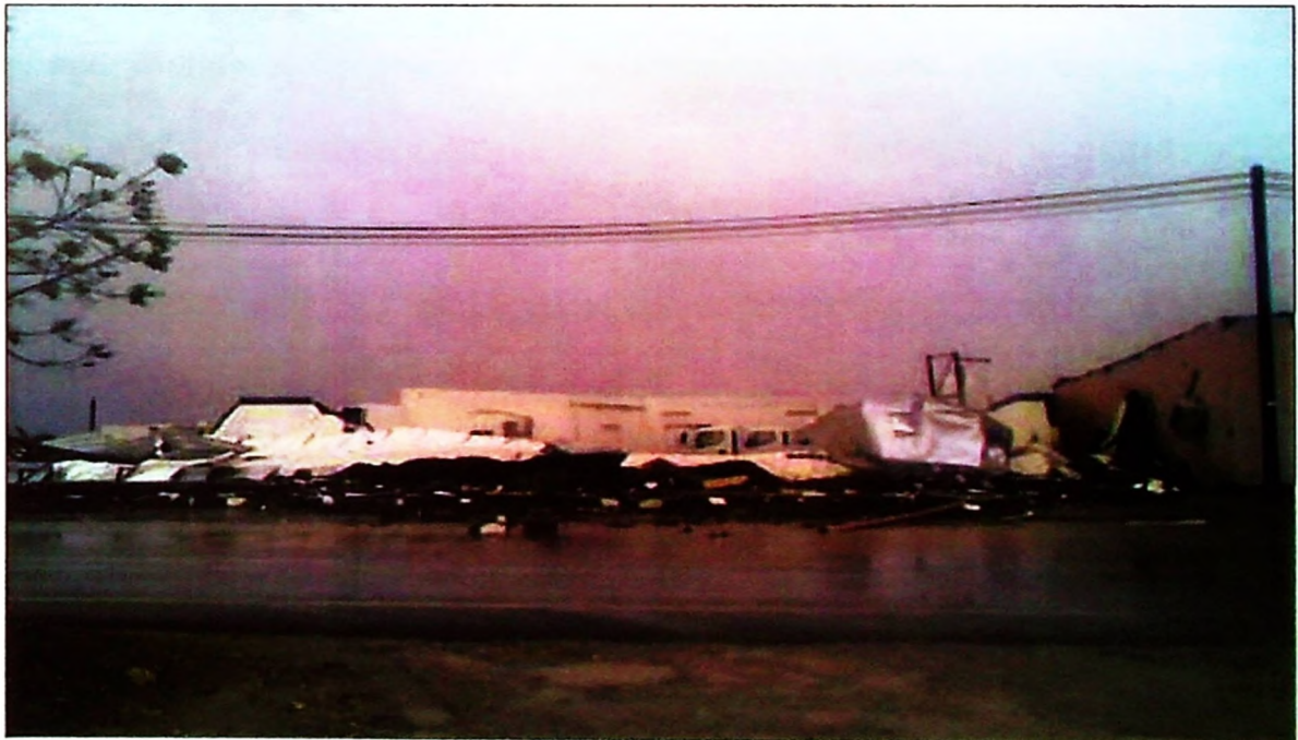
Figure 1.7: Damages caused by Cyclone Phet (Roohoman, 2010)
