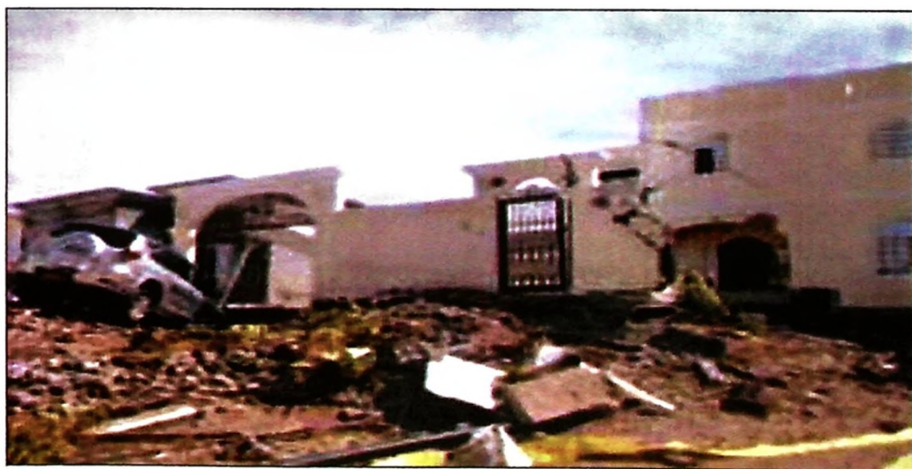
Figure 1.4: Damages in some houses caused by Cyclone Gonu (Roohoman, 2010)
