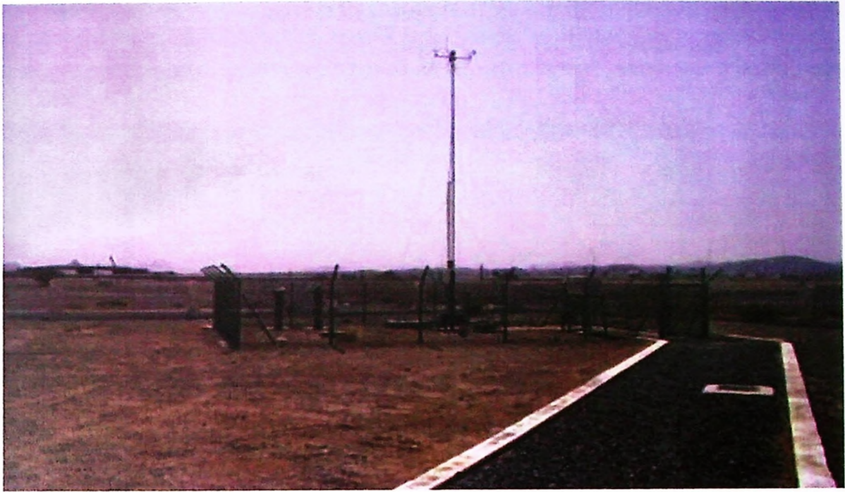
Figure 2.2: Wind speed measuring station at Nizwa
