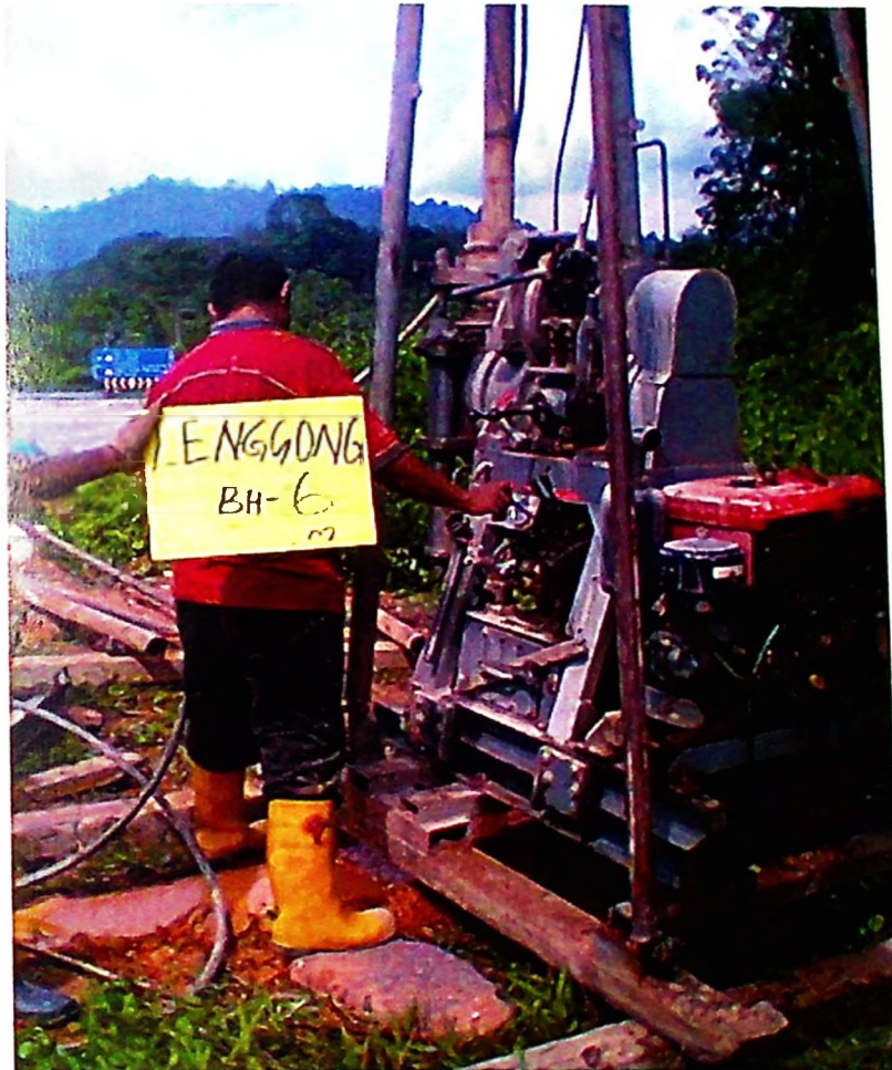
Boring (BH 6) work in progress at Bukit Bunuh, Perak.
