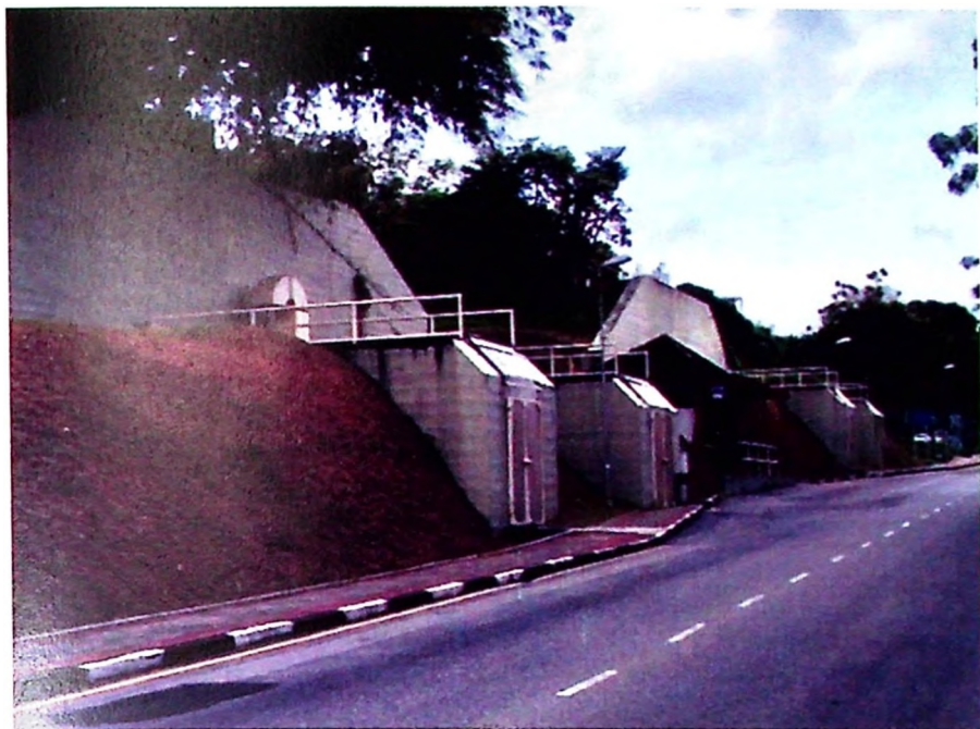
View from outside the buried bunker (Field model).
