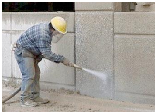
Figure 2.1: Abrasive blasting operation (Abrasive blasting: Know the hazards, 2017).
