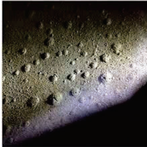
Figure 2 A failed metal structure with blisters found on the surface.
