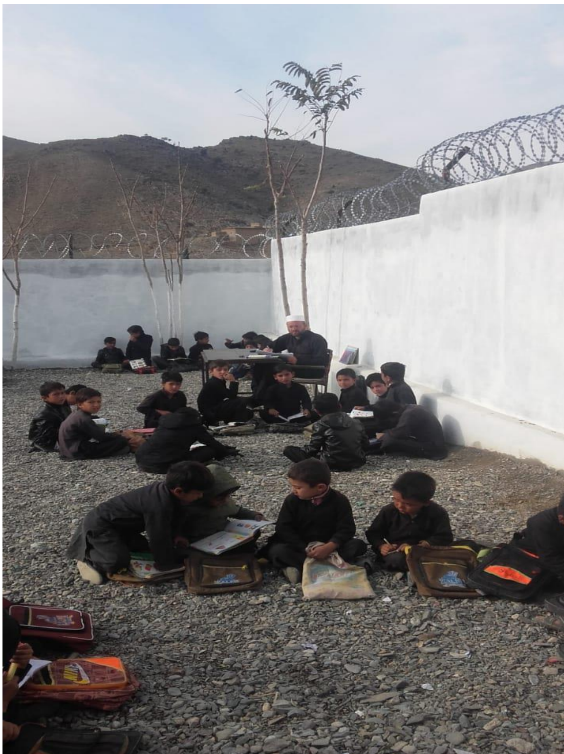
Figure 1.11 Dilapidated Condition of Govt. Boys Primary School, Bazar Zakha Khel, District Khyber Agency, Pakistan
