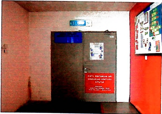
Figure A3.3: Picture of Main Door a.k.a Emergency Door
