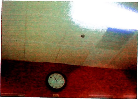
Figure A3.4: Picture of Water Sprinkler
