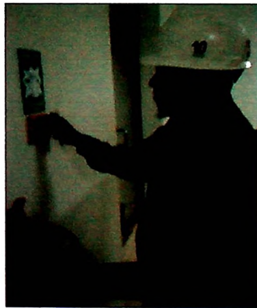
Figure A2.3: Picture of Testing for Fire Alarm
