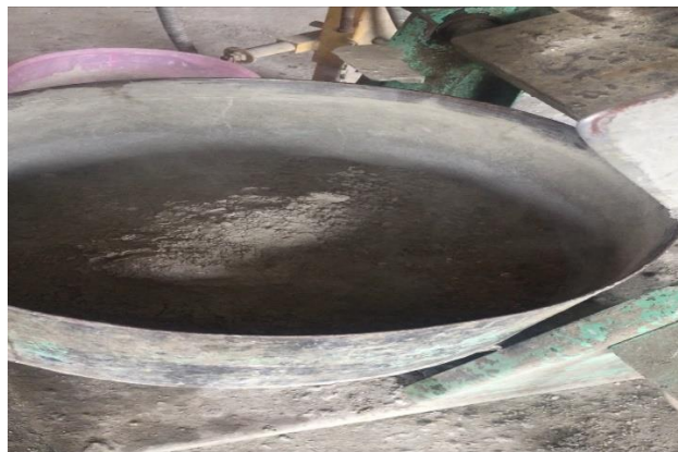
Figure 3.5: Dry mixing of concrete prior to addition of water
