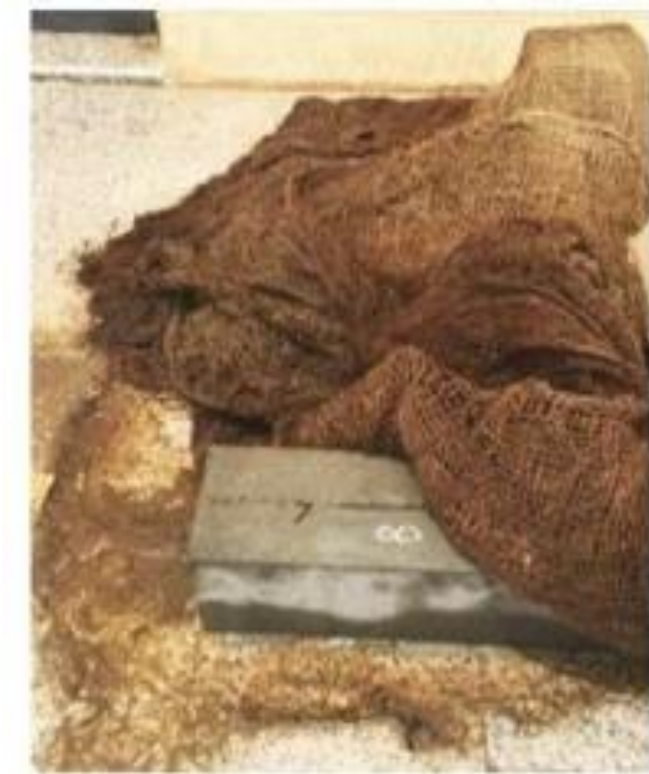
Figure 2.5: The curing of concrete structure with wet gunny curing (Zeyad, 2017)
