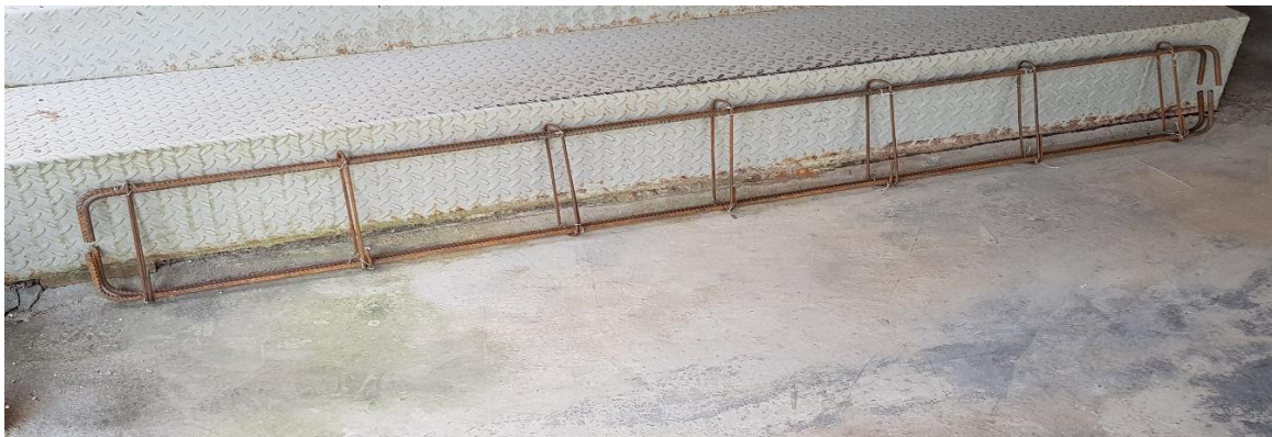
Figure 3.2: Completed reinforcement for beam (1 st set)
