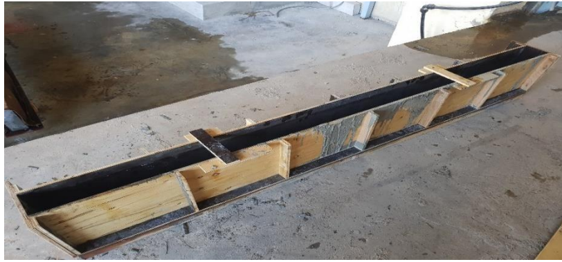
Figure 3.6: Beam Formwork (100mm x 300mm x 2000mm)
