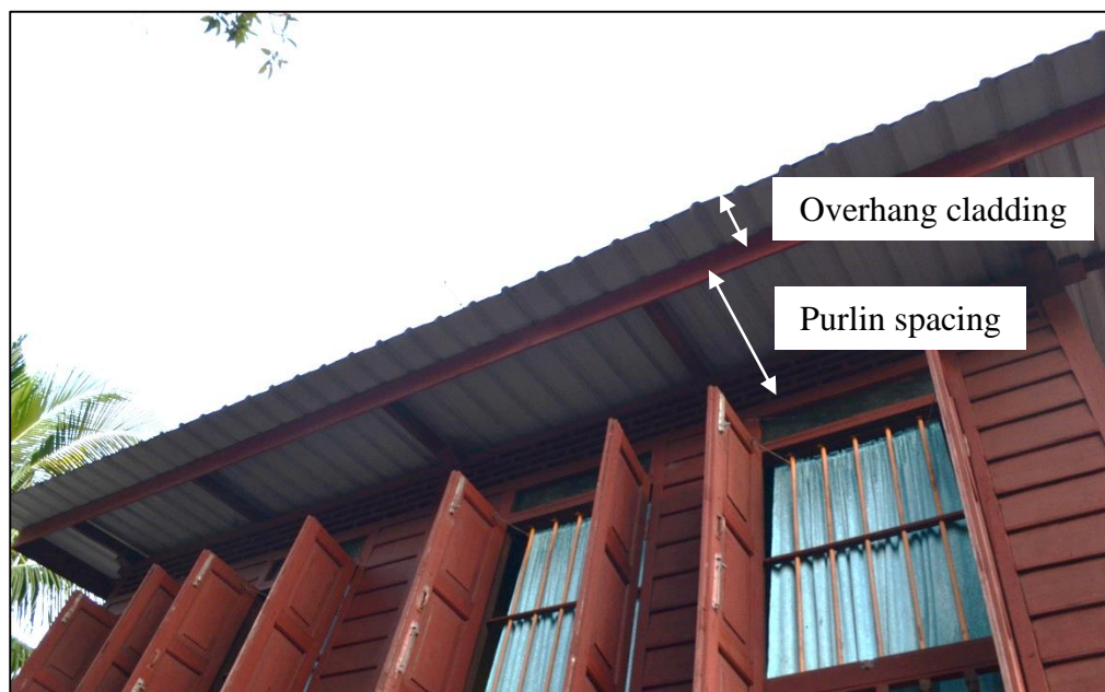
Figure 3.5 Part of overhang roof comprised of purlin spacing and overhang cladding
