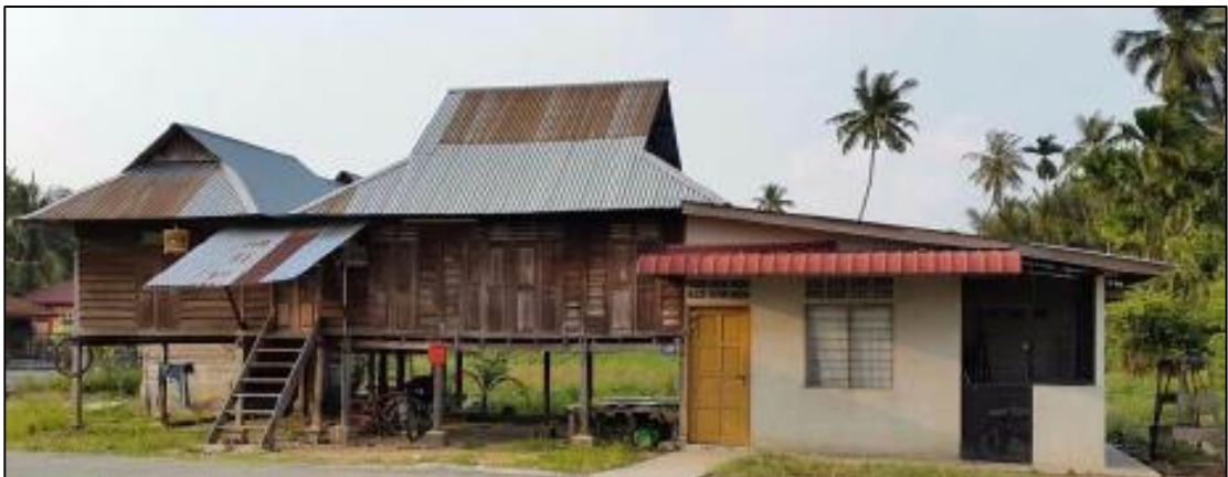
Figure 2.1 Typical house of rural area in Malaysia ( Muhammad et al., 2015)
