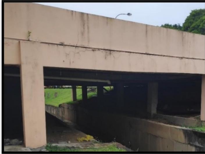
Figure 3.5 Location 3 – At a drain near PPSK buildings
