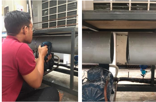
Figure 3.17: PVC pipe is removed using jigsaw
