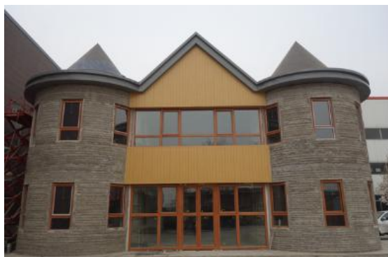
Figure 2.8: two-storey house built by Huashang Tengda [18]
