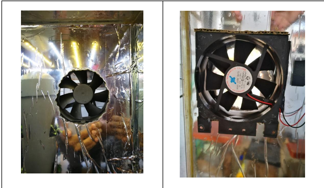
Figure 3.10: Fan Installation for Ventilation
