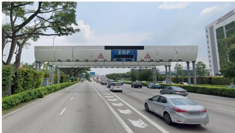
Figure 7 : Multi-Lane Free flow gantry
