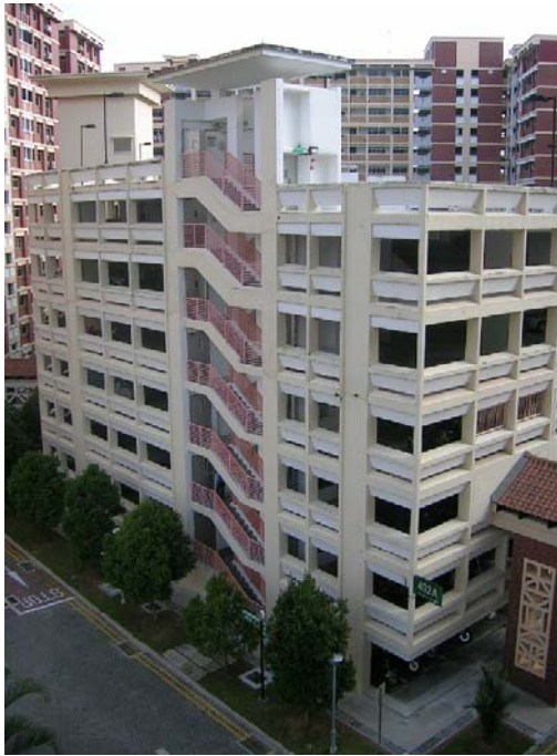
Figure 1.3: Multi-storey car park building
