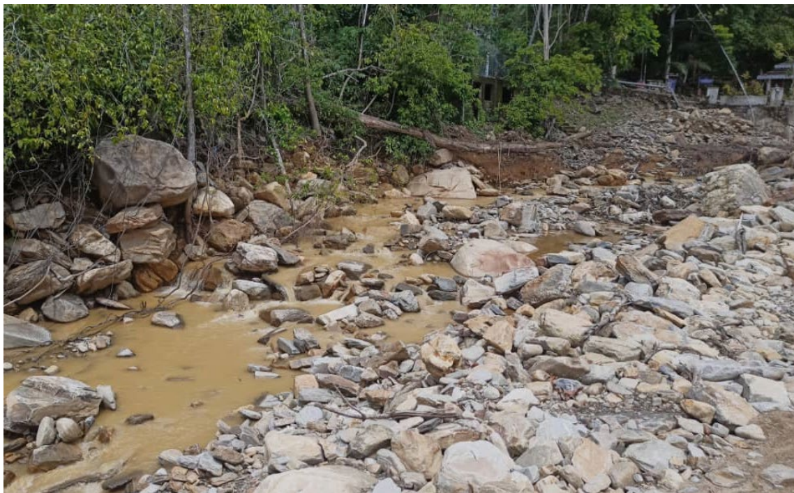
Figure 1.2: Mud and Debris Left on Site Near Titi Hayun, Gunung Jerai (Captured on 17 th March 2022)
