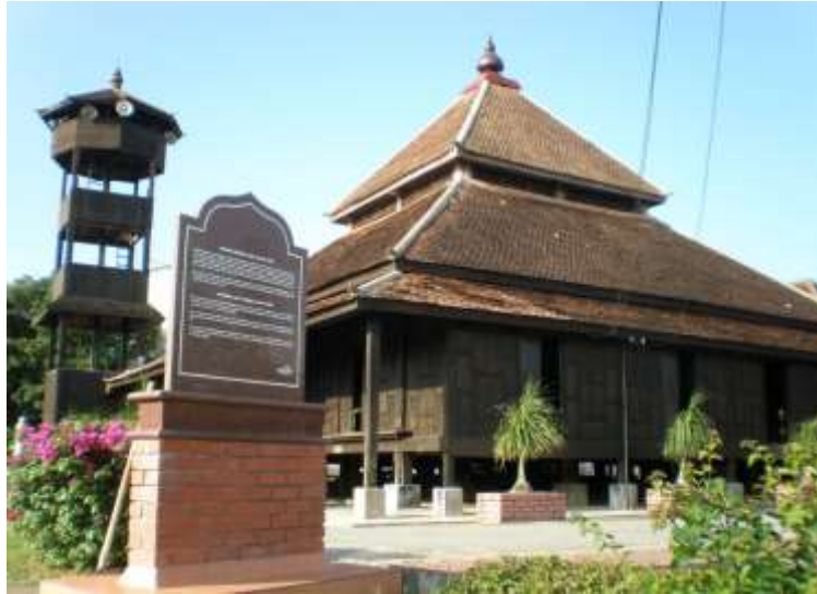
Figure 2.3: Kampung Laut Mosque in Kelantan (pyramidal-shaped roof)
