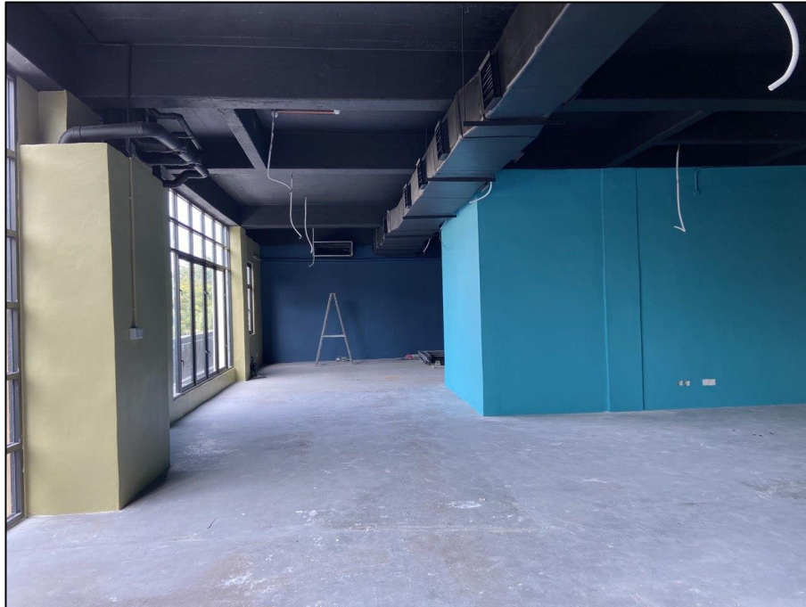
Figure 3.3: Tetupai Lounge during renovation
