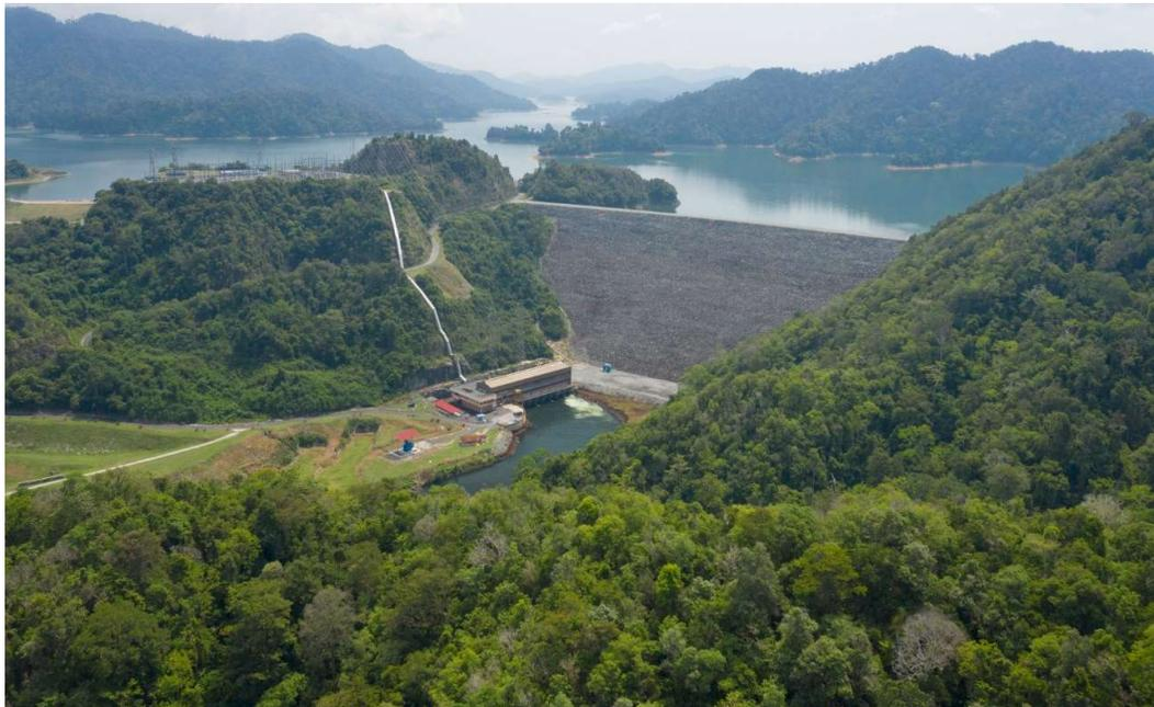
Figure 2.3: Rockfill dam – Temenggor Dam
