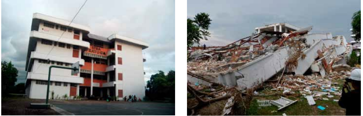
Figure 1.2: Before and after pictures of 4-story school building in Padang City, Indonesia (EERI, 2009)
