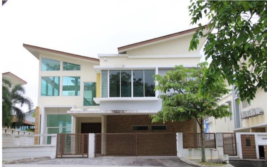
Figure 2.2 House with butterfly roof
