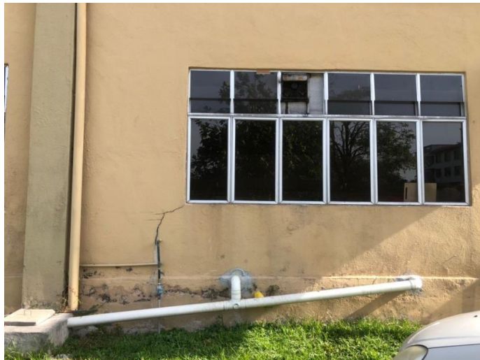
Figure 3.2 The wastewater sampling at behind Café Haleem Lembaran
