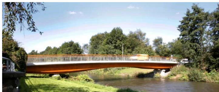
Figure 2.9: Agger TCC bridges in Germany (Holzindustrie, 2018)
