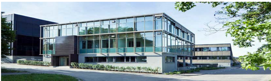
Figure 2.11: Four storeys ETH house of Natural Resources (Frangi et al., 2014)
