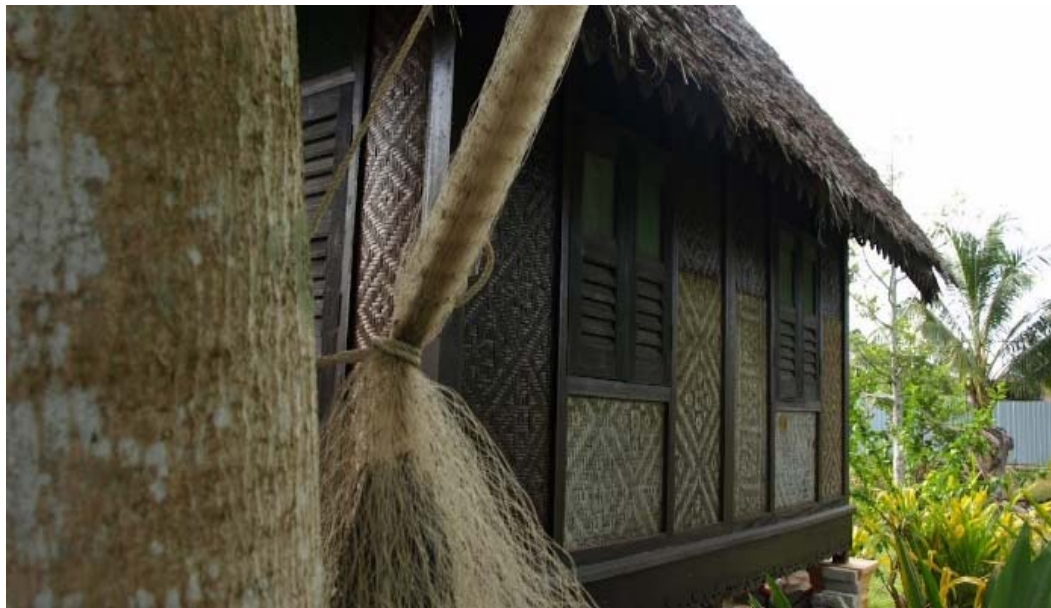
Figure 1-2: Exterior wall made of bamboo (Photo adapted by the author from Google Image)
