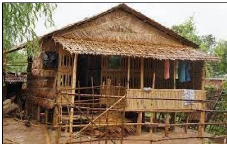
Figure 1: Traditional construction in Burma, Myanmar (Mertens & Audrey, 2019)
