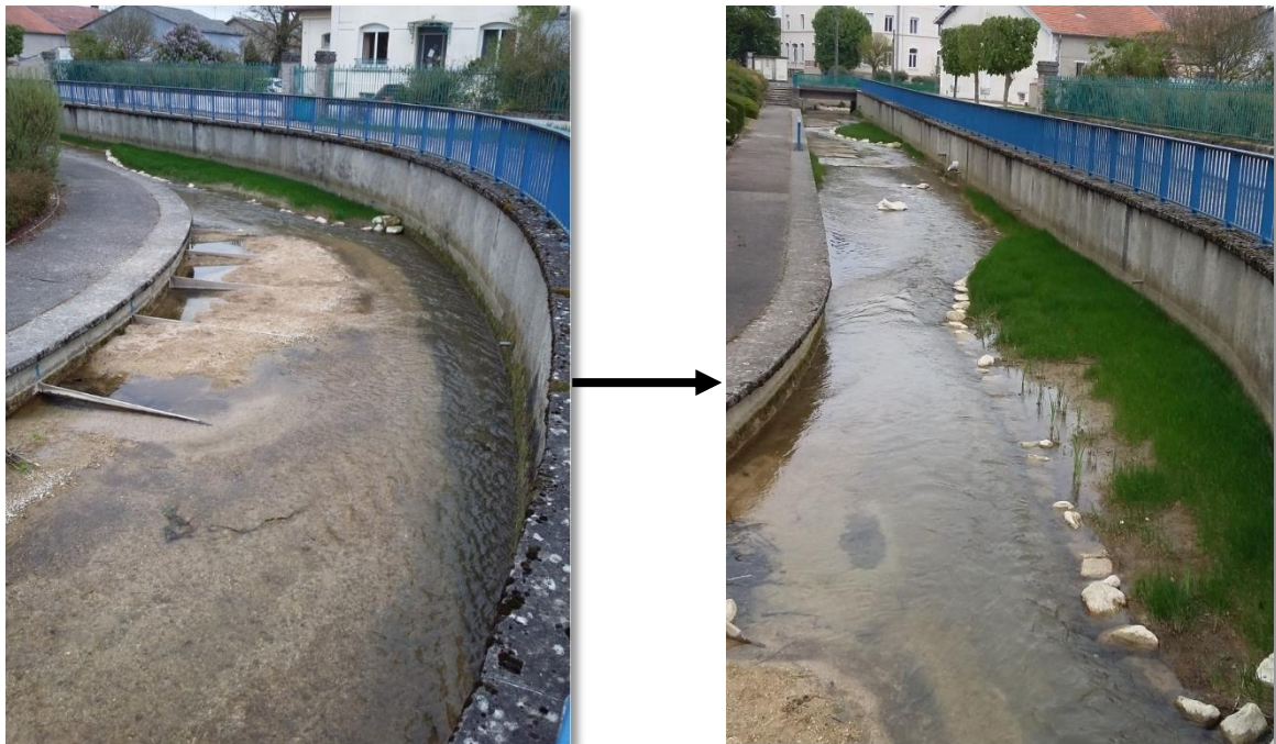
Figure 2.3: Application of spur dike to induce sand bar formation for storm drain improvement in Fresnes-en-Woevre, France (Pansera Jean-Noël, 2018)
