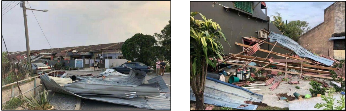
Figure 1.1 Examples of roof uplift of low-rise house in Ipoh, Perak (The Star,2022).
