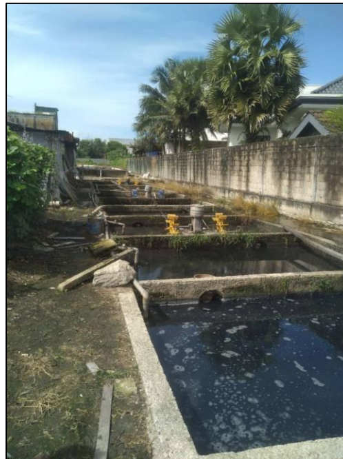
Figure 2.2: Lagoon treatment system at one of the pig farms in Kampung Selamat
