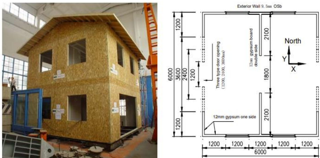
Figure 2.2 Full size two-storey timber model and main floor plan dimensions (Haijiang et al., 2008)
