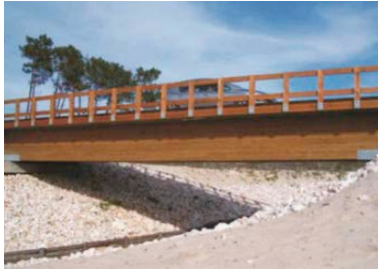
Figure 2.2 (b): TCC bridge after construction (courtesy of A.M.P.G Dias, 2013)
