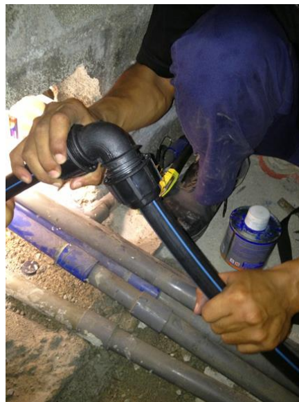
Figure 3.3 Pipe repair work is carried out
