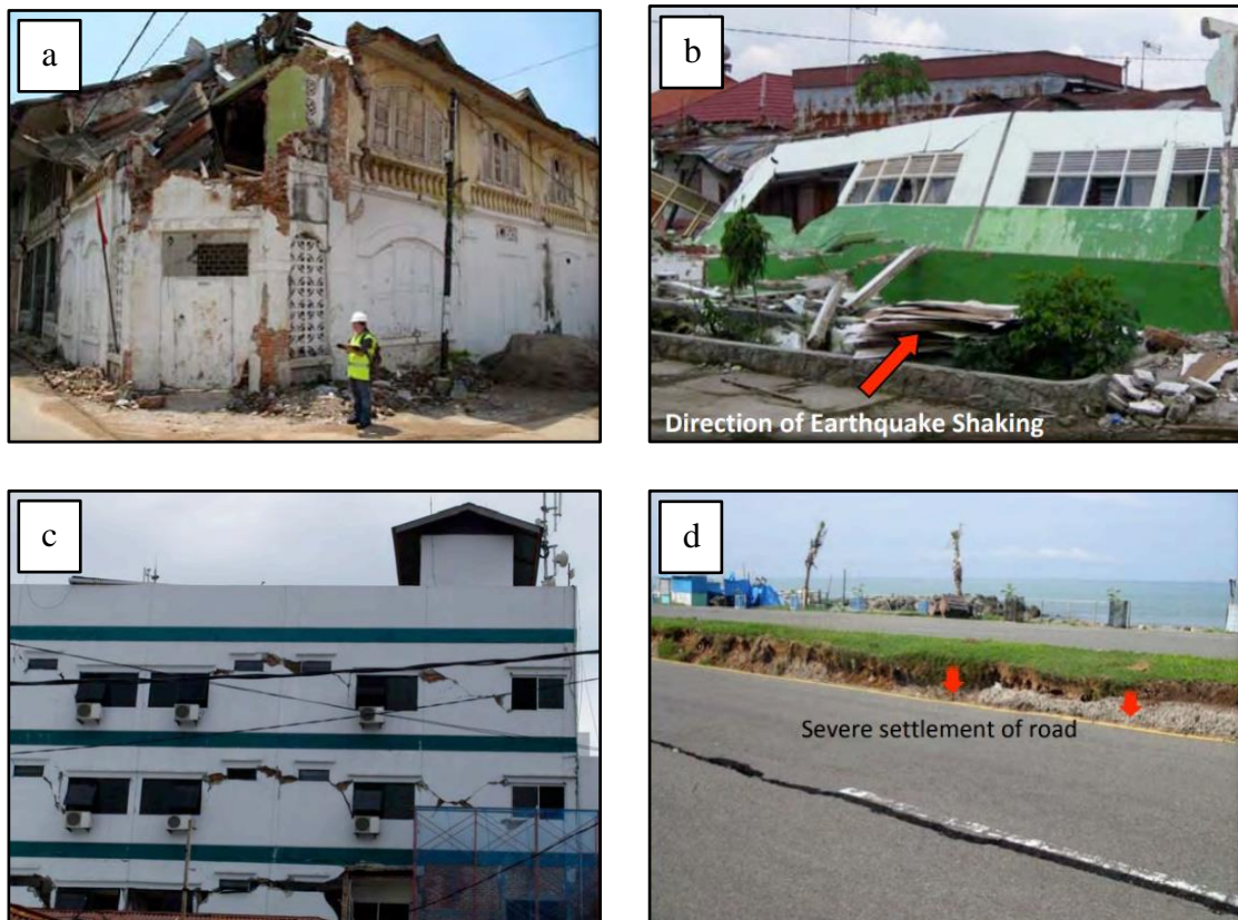
Figure 1.2: (a) Damaged house (b) Collapsed of school (c) Extensive cracks (d) Settlement on the roadway (Wilkinson et al., 2009)
