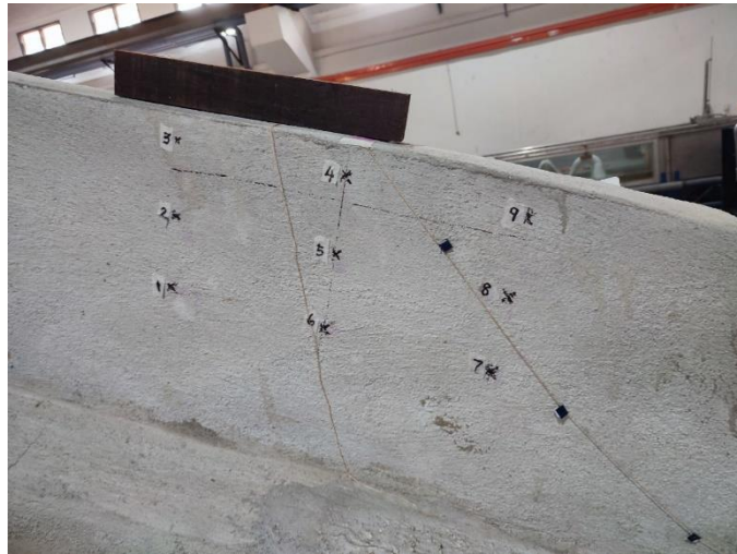
Figure 2.8: Vibration Analysis measurement points in Spillway section
