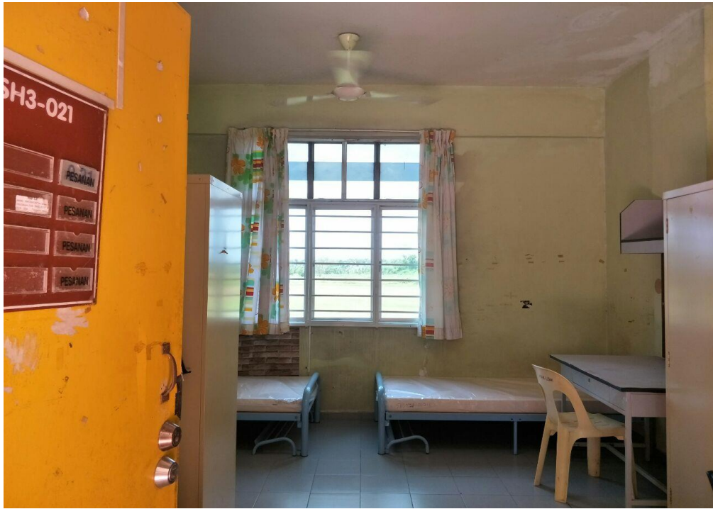
Figure 3.3 The overview of student dormitory
