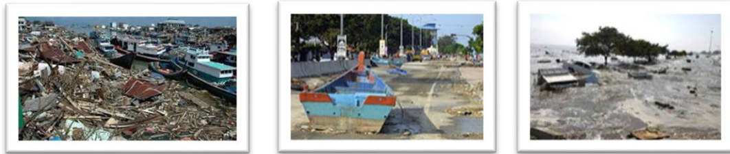
Figure 1.1: Damaged from Indian Ocean Earthquake 2014 (MinDef, 2019)
