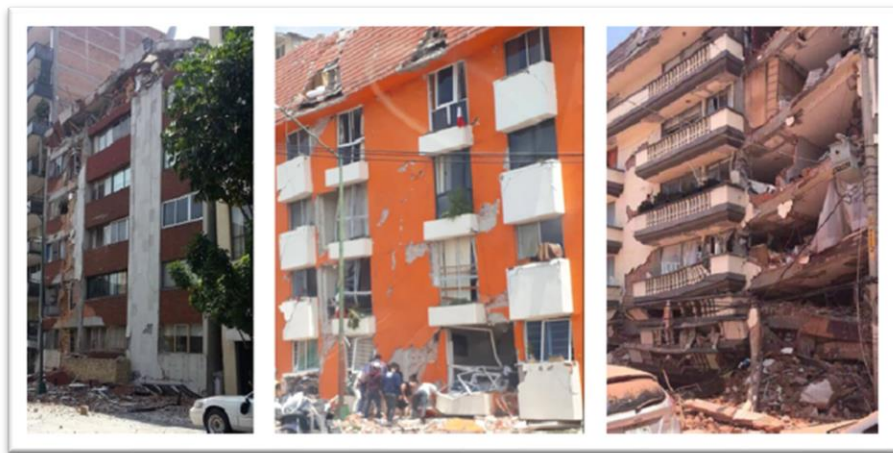
Figure 2.2: Collapse of the building in Mexico City (Jara et al. , 2020)
