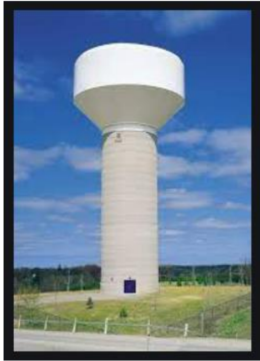
Figure 2-4 : Pedestal Elevated Water Tank.
