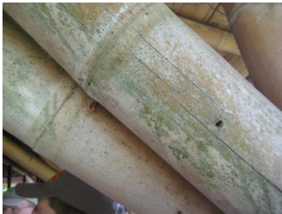
Figure 2. 4 Visible exit holes due to beetle damage (Kaminski et al., 2016)
