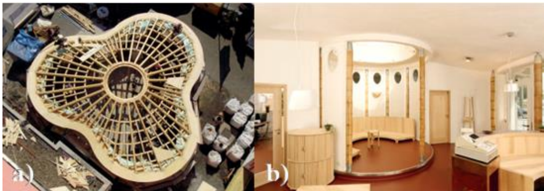
Figure 2. 8 (a) Timber roof construction and (b) bamboo columns in an office building, Germany (Minke, 2016)
