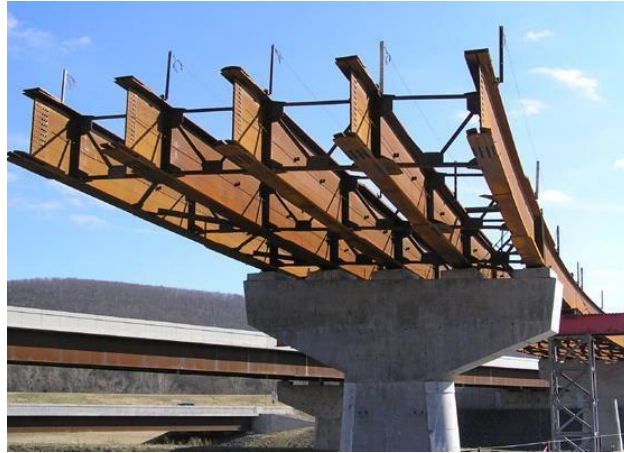
Figure 2. 5: The plate girder bridge (Ehab E. 2014)
