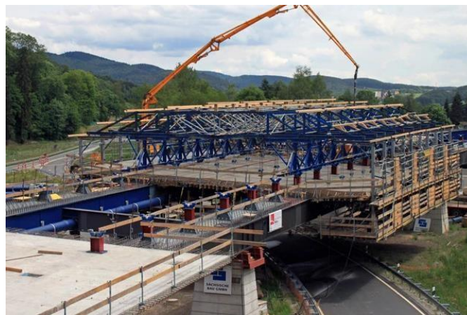
Figure 2. 6: The slab casting on steel girder bridge (Ehab E. 2014)
