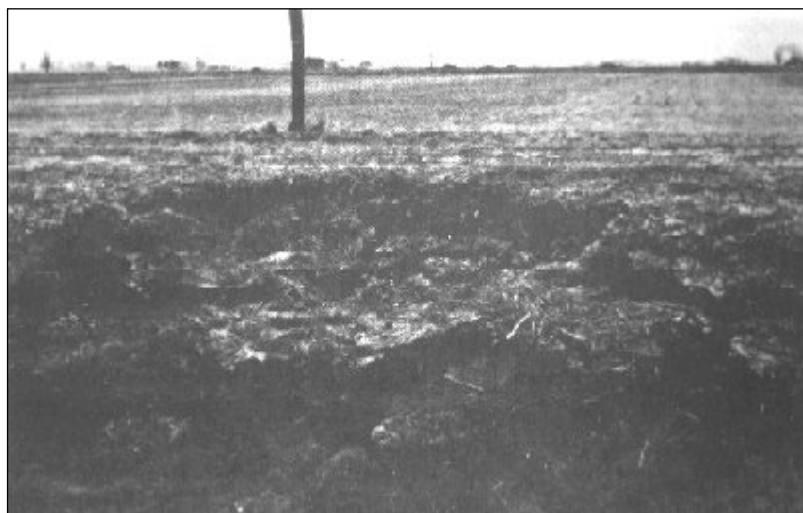
Figure 2.3: Stream and Ditch Bank erosion
