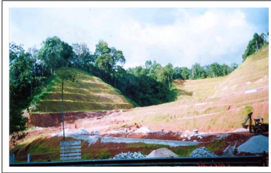
Figure 2.10: Usage of plants as a soil cover material on the surface of escarpments
