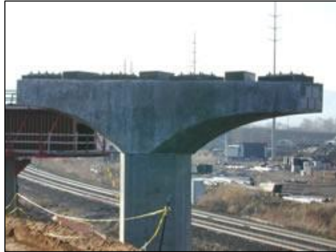
Figure 1.1: Hammerhead Bridge Pier (United Forms Corporation)
