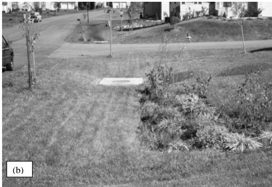
Figure 2.5 (a) Highway median bioretention, and (b) Swale-side bioretention system (Retrieved from The Prince George's Country, 2009).
