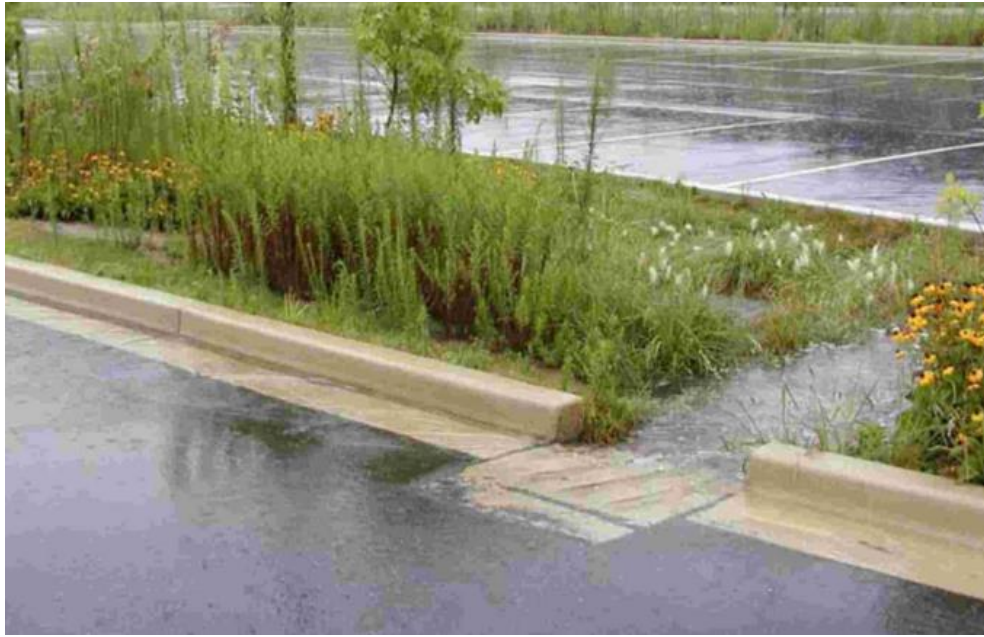
Figure 2.3 Showing the bioretention facility installed at a parking lot (Retrieved from Davis et al., 2009).
