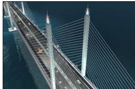
(b) Penang Second Bridge in Pulau Pinang, Malaysia
