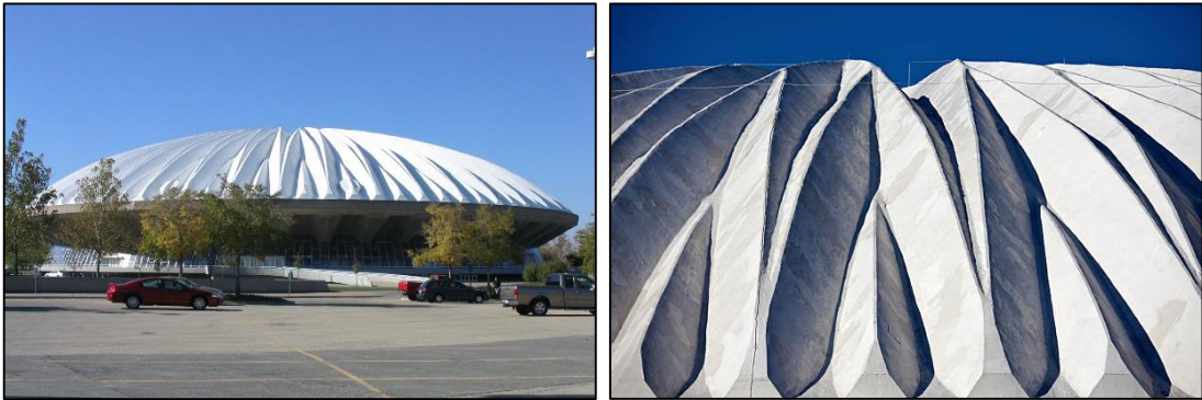
(b) State Farm Center in Illinois, USA (Dori, 2003, Benkrut, 2013)
