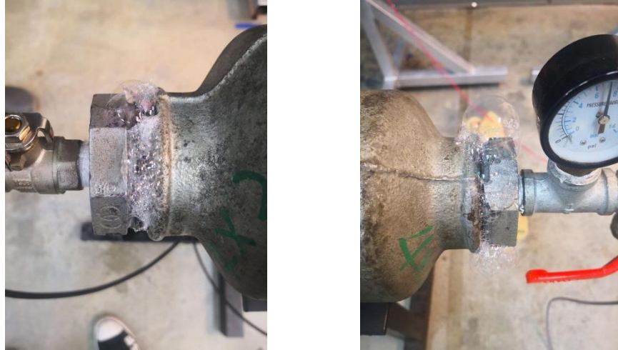
Figure 3.3: Gas leaking is found on the pipe joint using visual inspection technique
