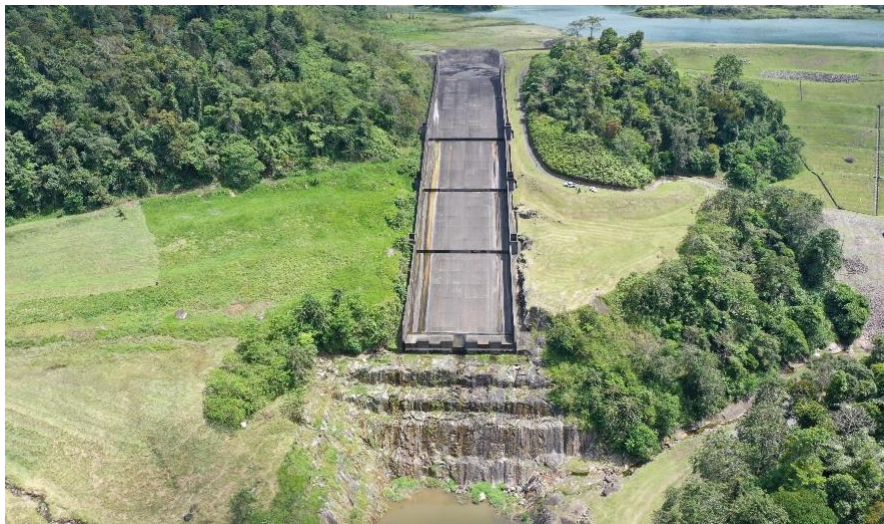
Figure 1-1: Drone View of Pergau Spillway
