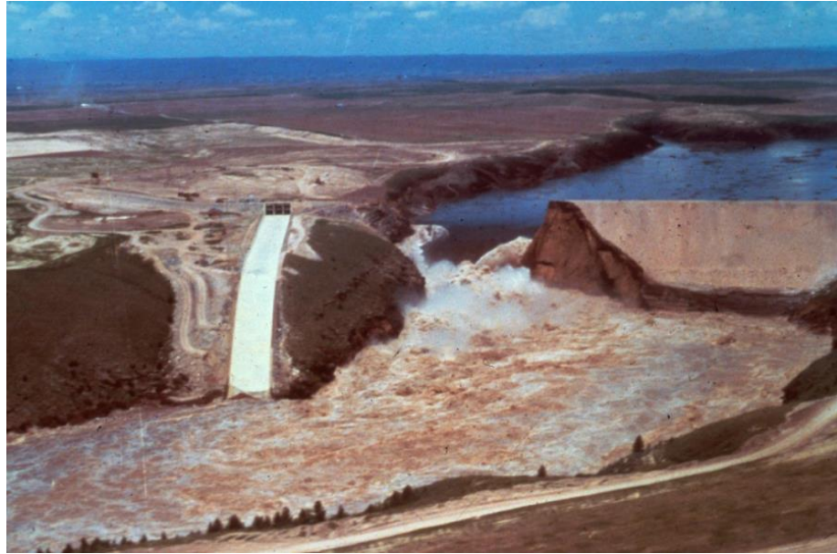
Figure 2-1: Teton Dam failure
